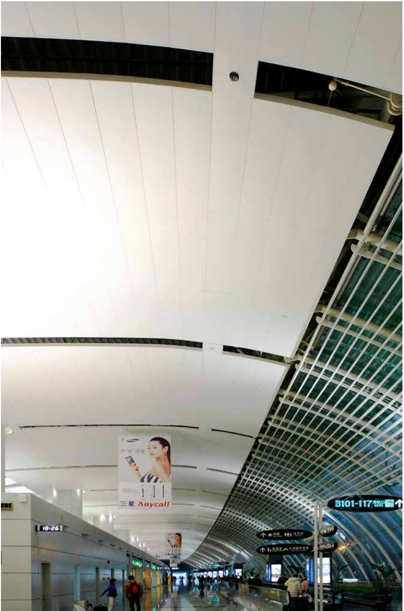
Project: Guangzhou Baiyun International Airport, China - Product: Luxalon® 300C Wide Panel Ceiling Architect: Parsons Technology Group Corporation & URS Greiner & Architectural Design & Research Institute of Guangdong Province
