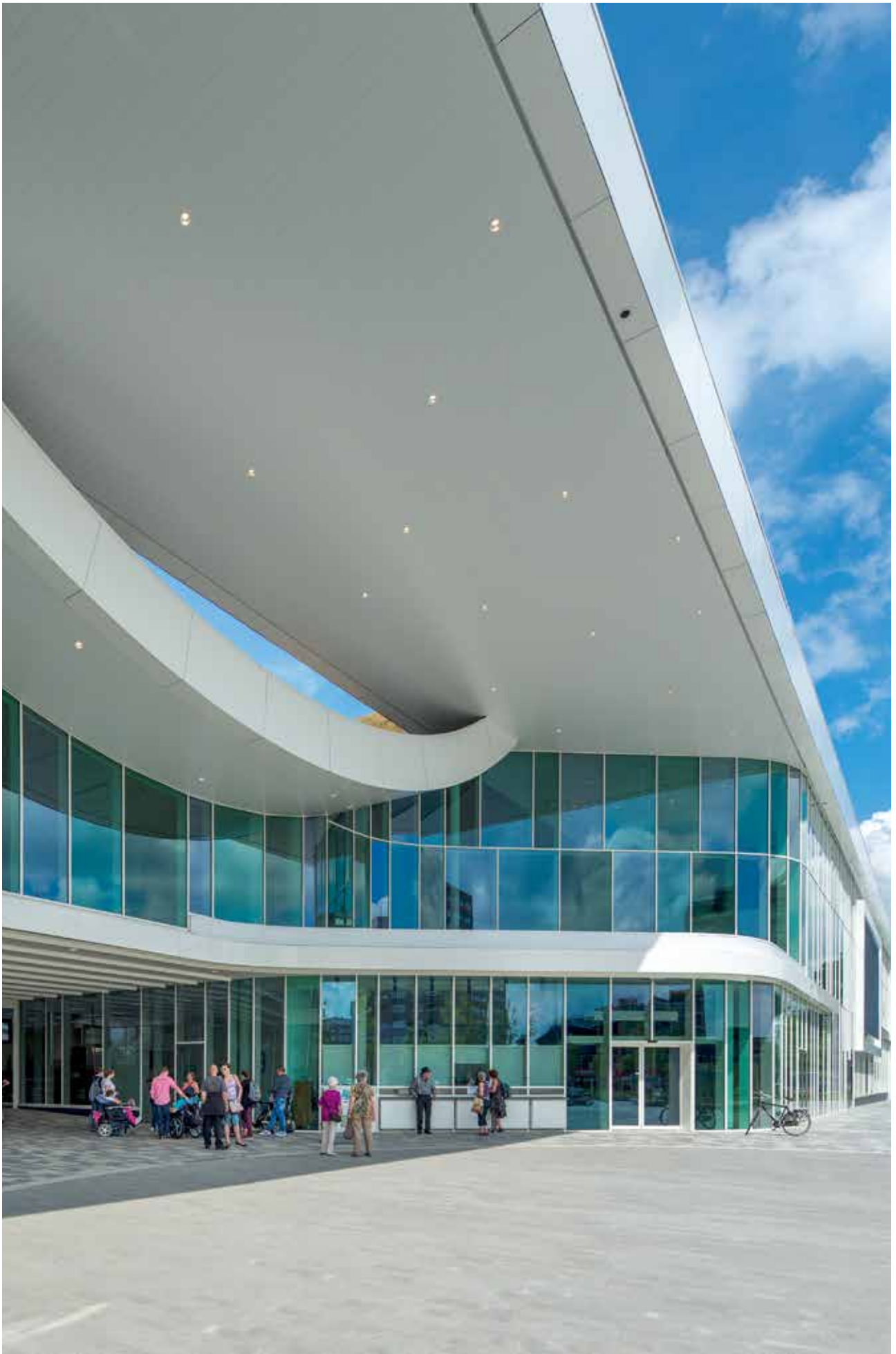
Project: Wildlands, Emmen, The Netherlands - Product: Linear 150F/200F - Architect: LKSVD architecten
