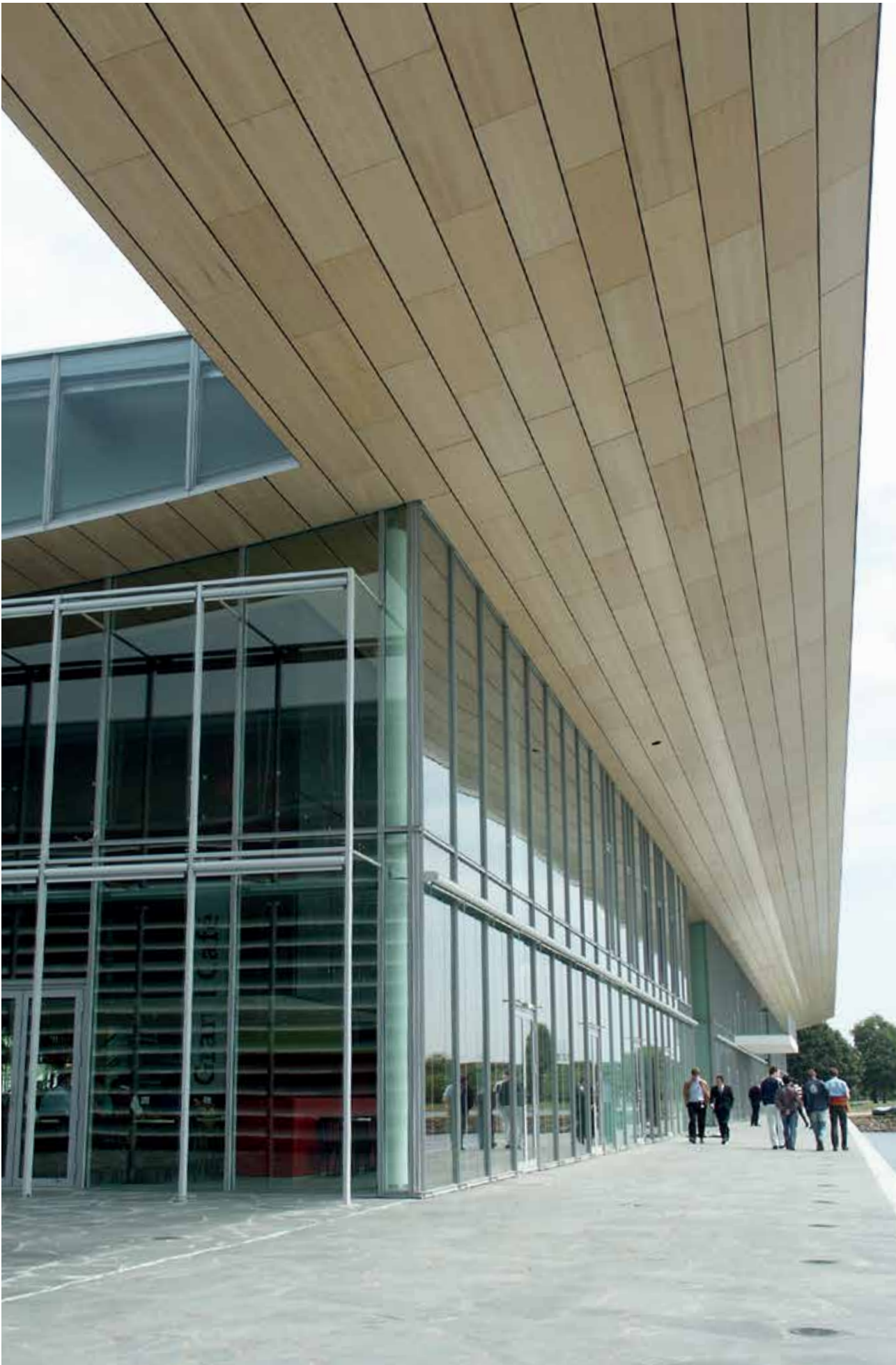
Project: Philips High Tech Campus, Eindhoven, The Netherlands - Product: Veneered Wood Tiles Exterior, American Maple - Architect: JHK Architecten
