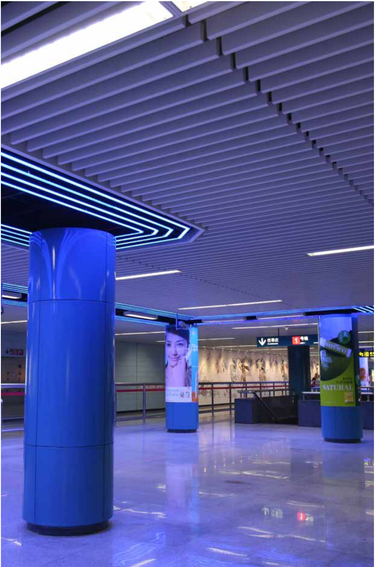
Project: Shanghai Metro Line 1, China - Product: Baffles Straight - Architect: Shanghai University Academy of Fine Arts
