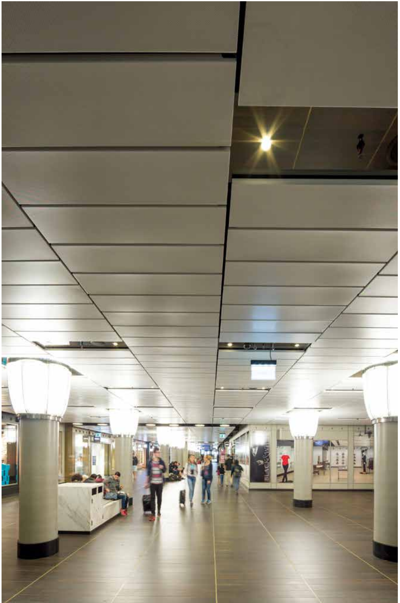
Project: Poortvrije Passages Amsterdam, The Netherlands; Hook-On panels - Architect: Benthem Crouwel Architects / Powerhouse Company / Merk X
