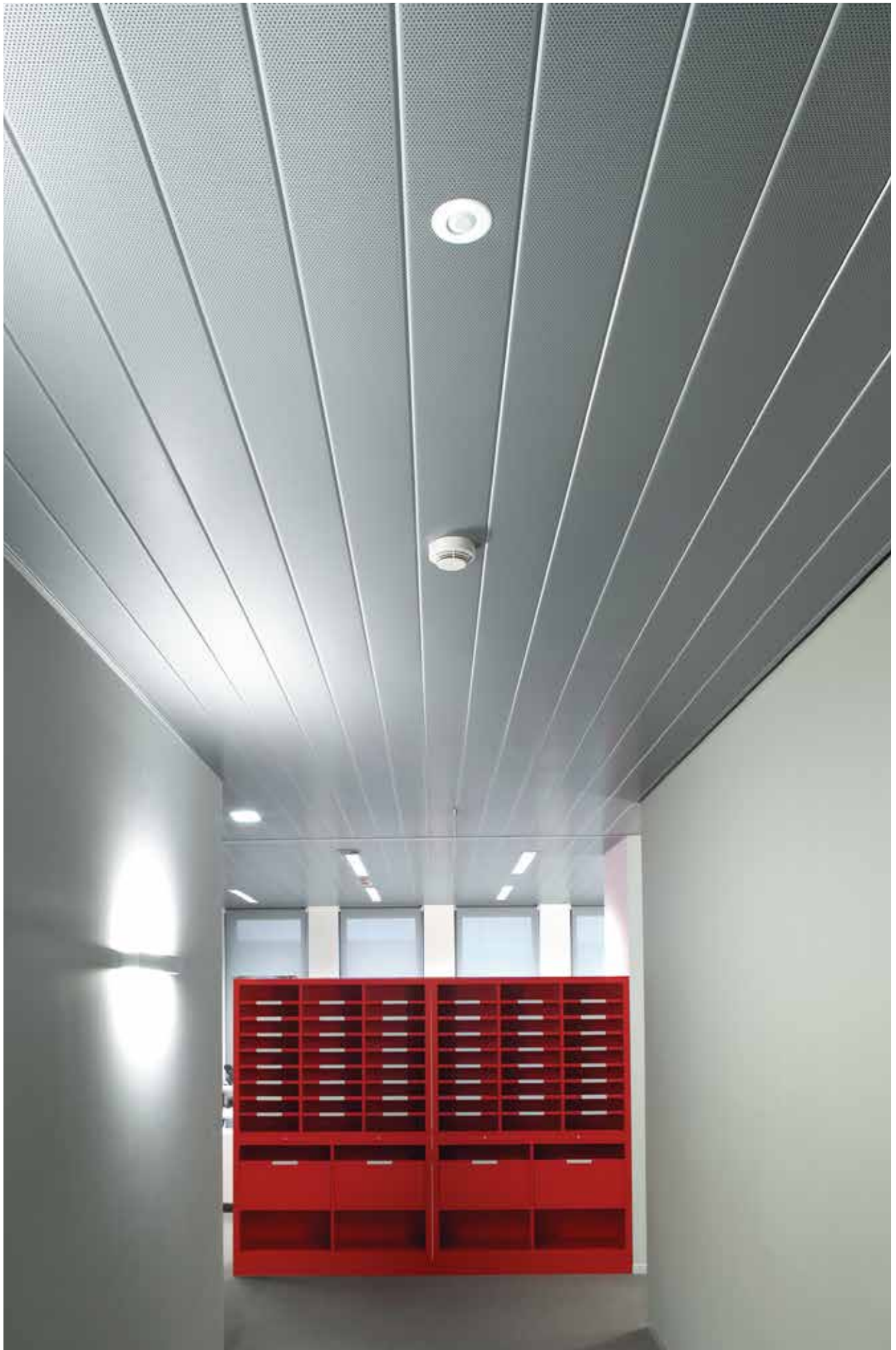
Project: InBev headquarters, Leuven, Belgium - Product: Linear 75C/150C/225C - Architect: Poponcini & Lootens
